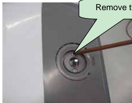
2. Remove two screws and remove temperature controller
